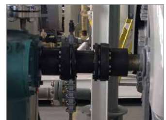
Rexnord® Thomas Disc Coupling hub mounted to water pump from motor using a TLK600 external locking device
